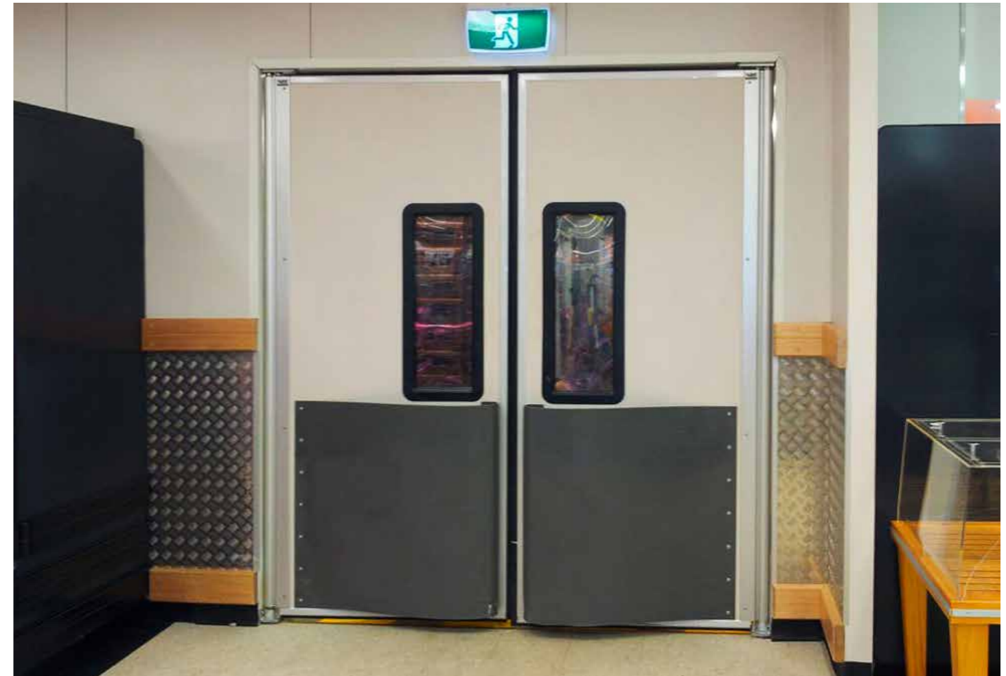
Double Action Door with Floor Spring
