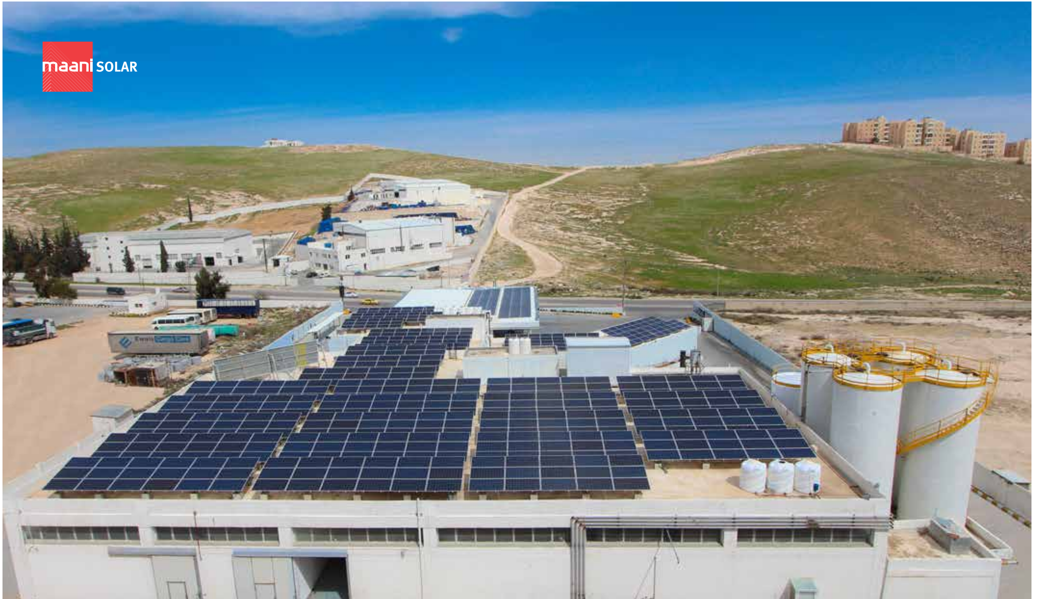
Title: Jopetrol National Paints Fuel Station Location: Amman, Jordan Scope: On-grid photovoltaic 210 kWp system
