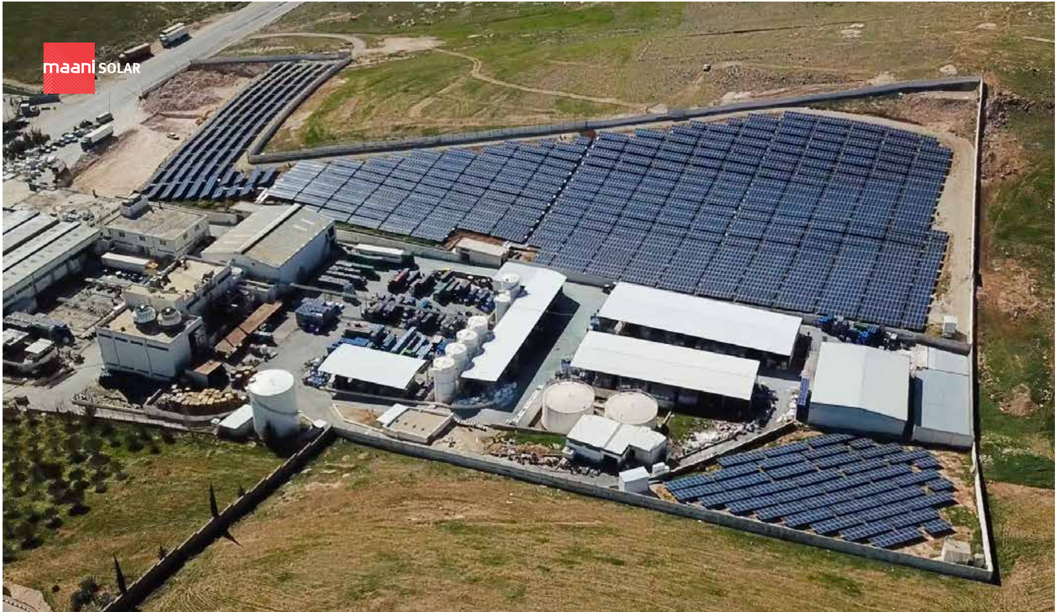
Title: National Paints / Sayegh Group Location: Abu Alanda, Jordan Scope: On-grid photovoltaic 2,809 kWp system
