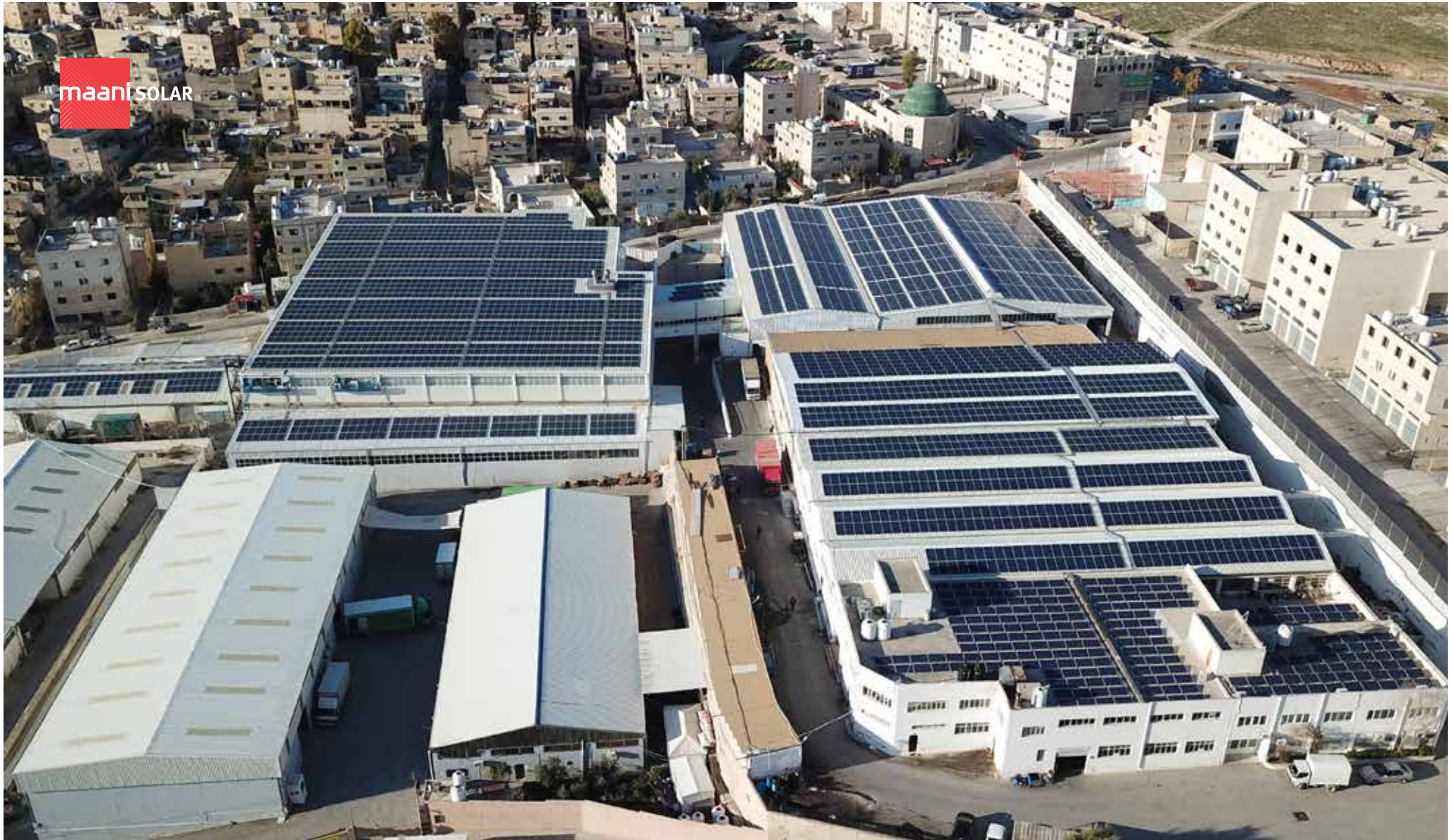
Title: Canning Industries Co. / Sayegh Group Location: Marka, Jordan Scope: On-grid photovoltaic 1,100 kWp system
