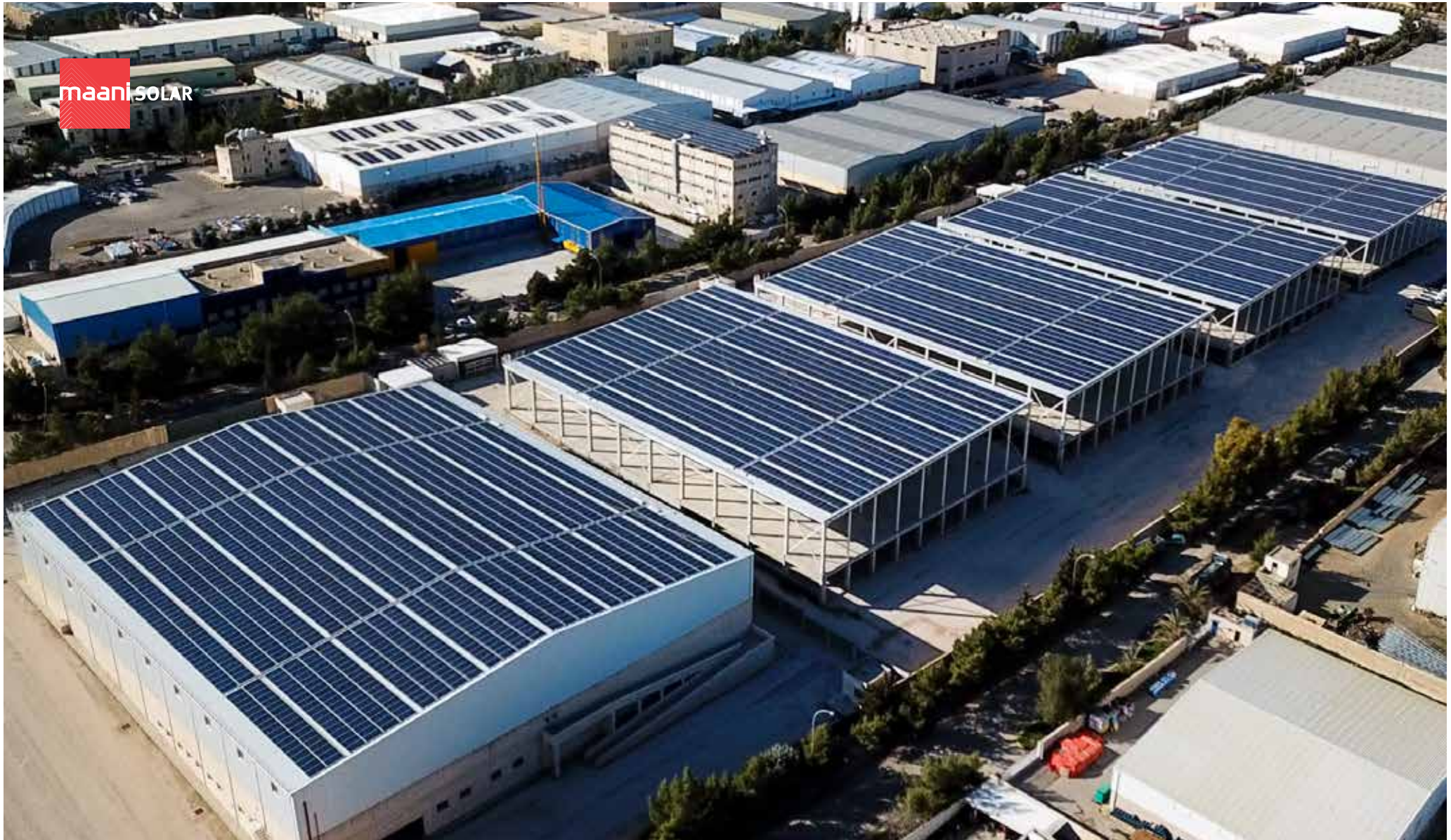
Title: Jordan Islamic Bank – (Bonded/Sahab) Location: Sahab, Jordan Scope: Wheeling photovoltaic 2,714 kWp system
